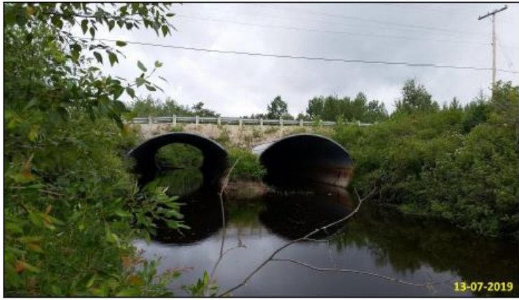
Picture 4 – East Elevation
