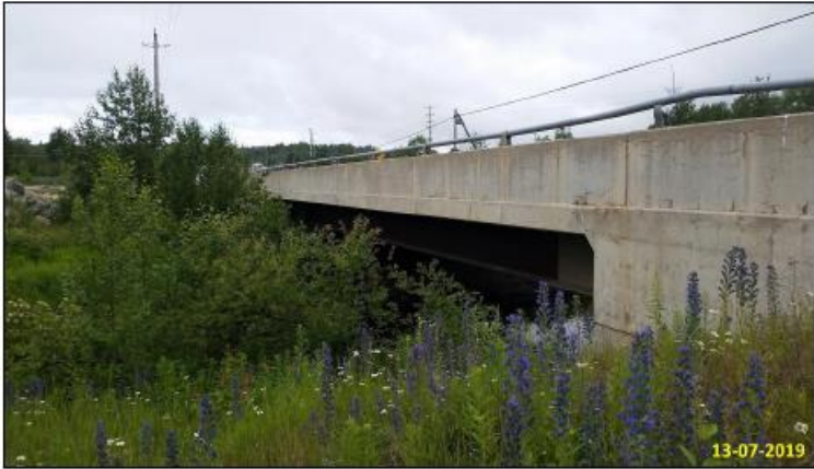
Picture 3 – South Elevation
