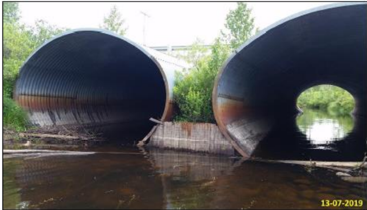
Picture 3 – West Elevation
