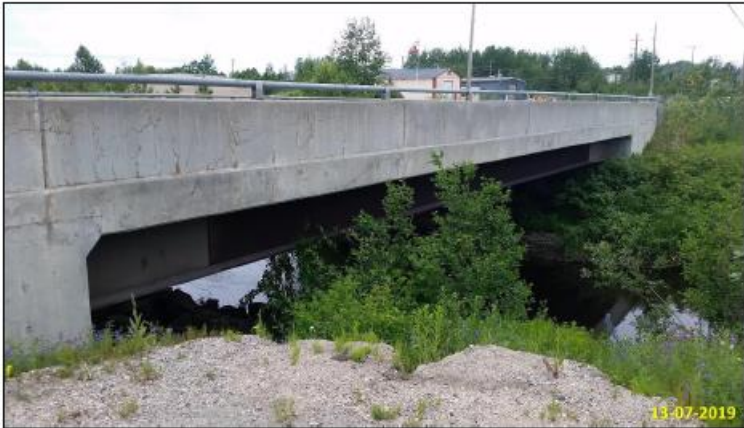
Picture 4 – North Elevation
